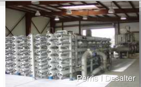
Hemet Water Filtration Plant
