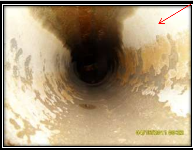
AC PIPE IN GOOD CONDITION
