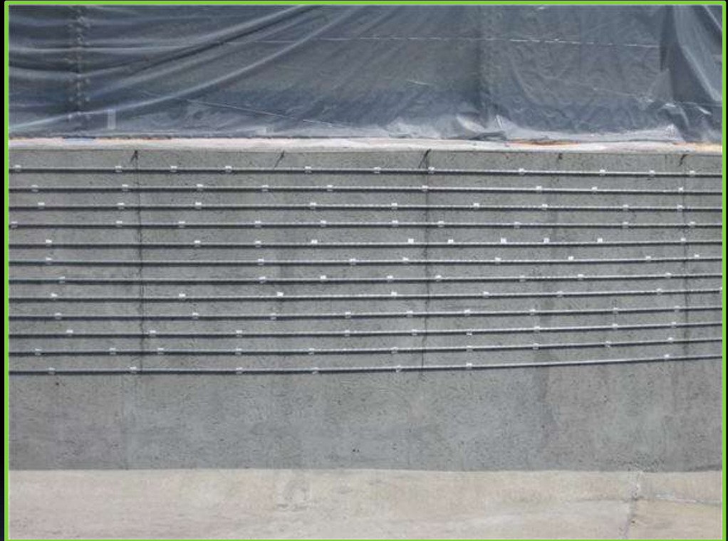
0.6 diameter galvanized cables installed with friction pads, ready for stressing
